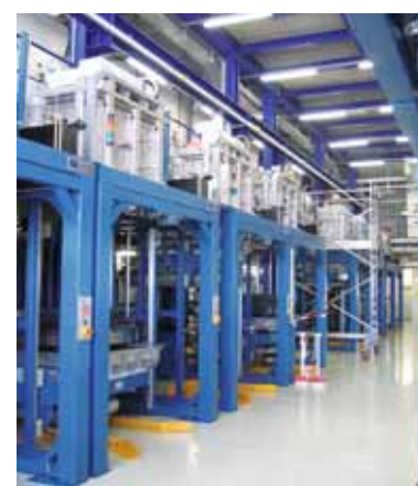
Fig. 1 View into a production hall with a number of identical "quasi-continuously operating high-temperature sintering furnaces"
